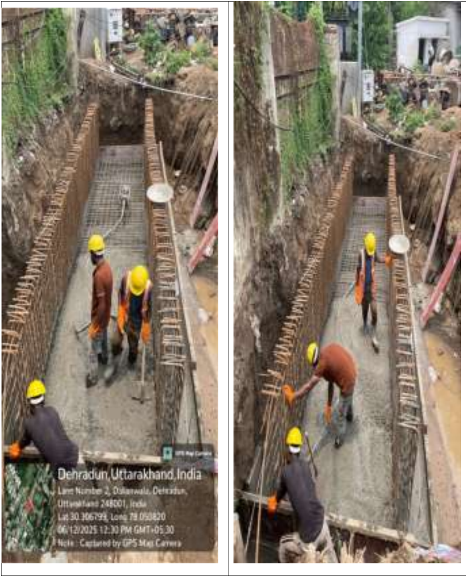
Labours equipped with proper safety gear
