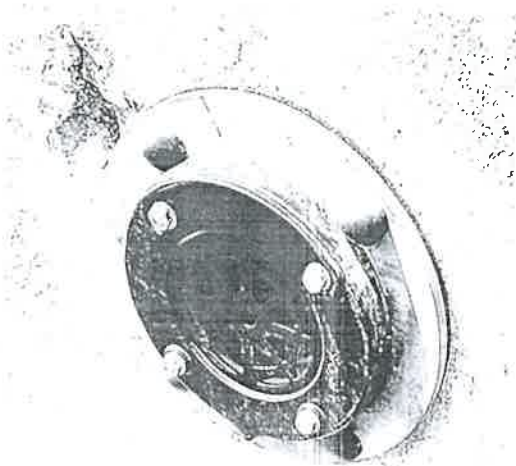
Fig.13. Fitting of readymade filter using bolts
